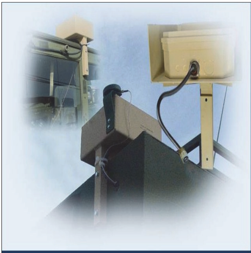
Figure 3-39. Inspect the MT 2011E Transceiver for cracks, and evidence of damage.
