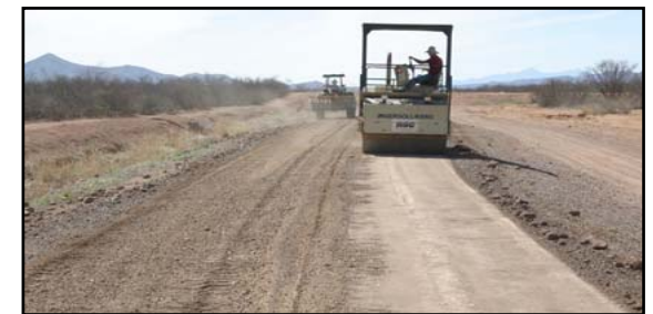
Figure 4. Compacting the Soil
