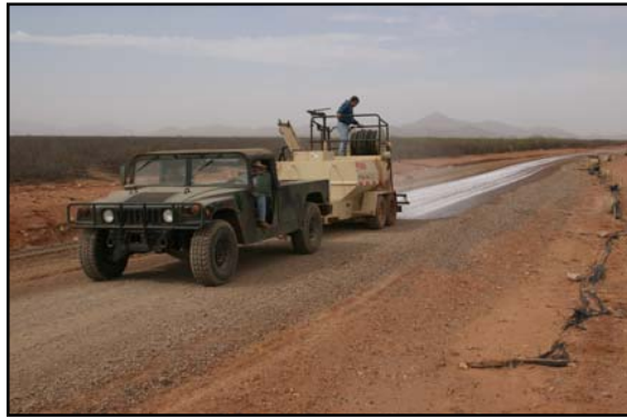
Figure 5. Spraying the Remaining Palliative
