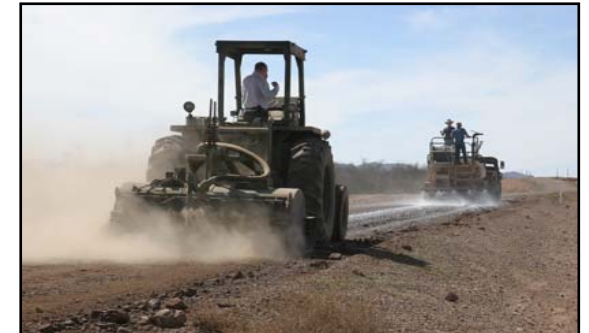
Figure 3. Spraying an Admix Application
