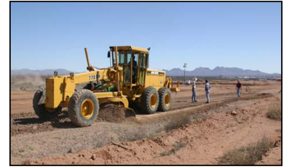
Figure 2. Grading the Soil
