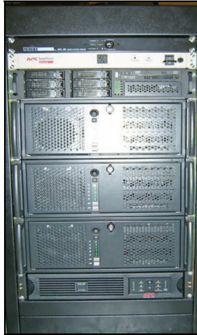
Figure 7-7. Instructor operator station (IOS) computer rack.
